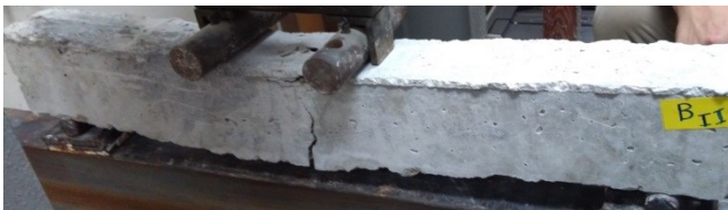
Fig. 14. crack pattern of control beam B II0
