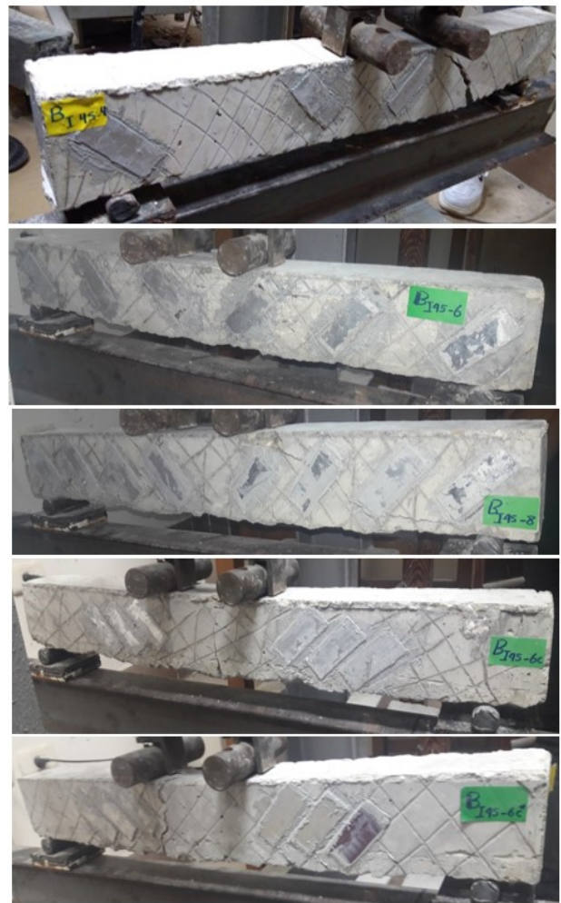
Fig. 11. crack pattern and mode of failure for the beams strengthen using strengthening technique (2).
