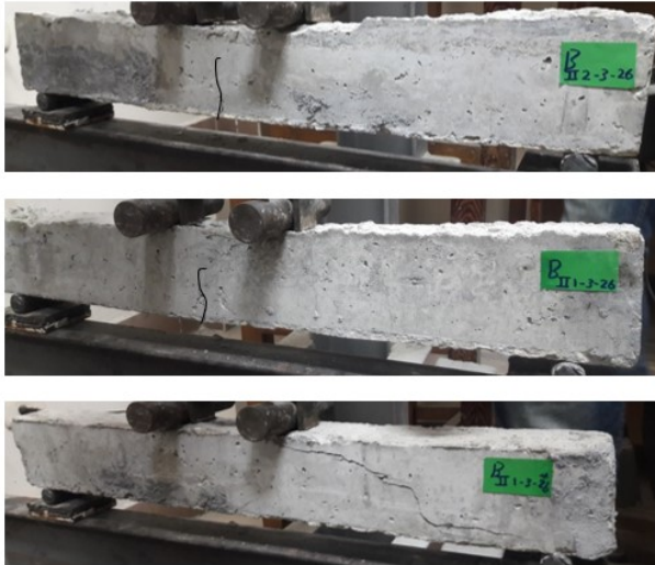
Fig. 16. crack pattern and mode of failure for the beams strengthen using strengthening technique (6).
